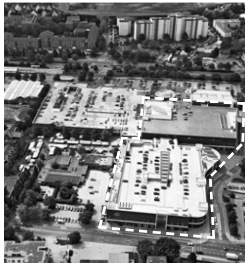
City Center, Langenhagen
