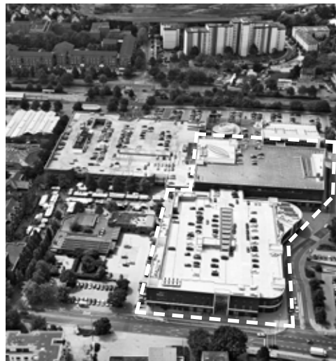
City Center, Langenhagen
